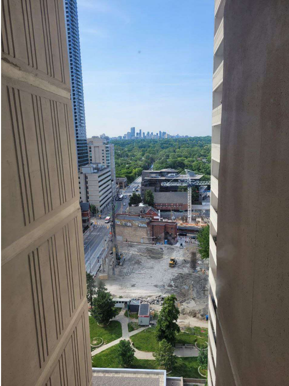
4) Two separate condo constructions on the stretch of 300m between St. James Town and Sherbourne Station. The view from the edge of St. James Town, to the North. In the front, relatively intact St. James Town West Park (photo taken in July 2023)
