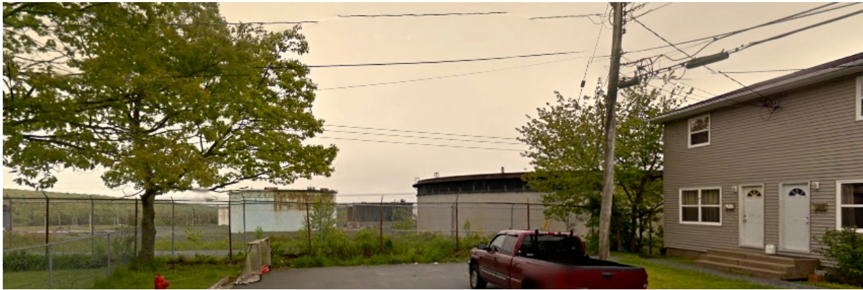
Figure 4.1.12 A view of the Imperial Oil Tank Farm from within South Woodside (Image taken from googol street view, November 15, 2014)
