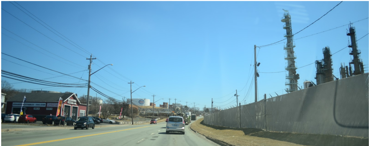
Figure 4.1.5 The view driving South on Pleasant Street in Woodside, with white privacy fence hiding the majority of the refinery
