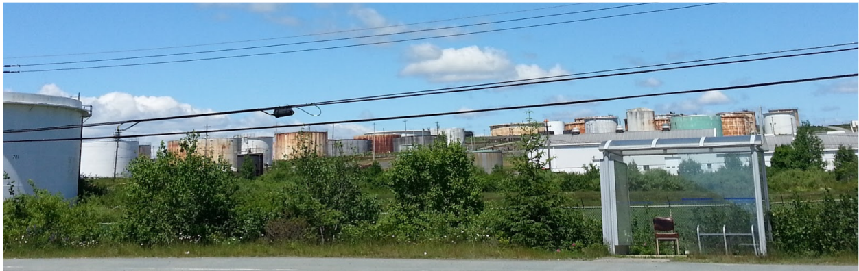
Figure 4.1.14 The rusting and unused Ultramar oil tanks, south on Pleasant Street in Eastern Passage
