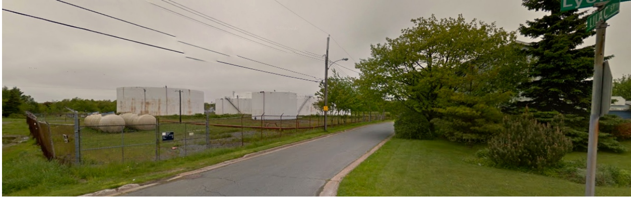
Figure 4.1.13 The Irving Oil tank farm, which is surrounded by houses within South Woodside (Image taken from Google Street View, November 15, 2014)
