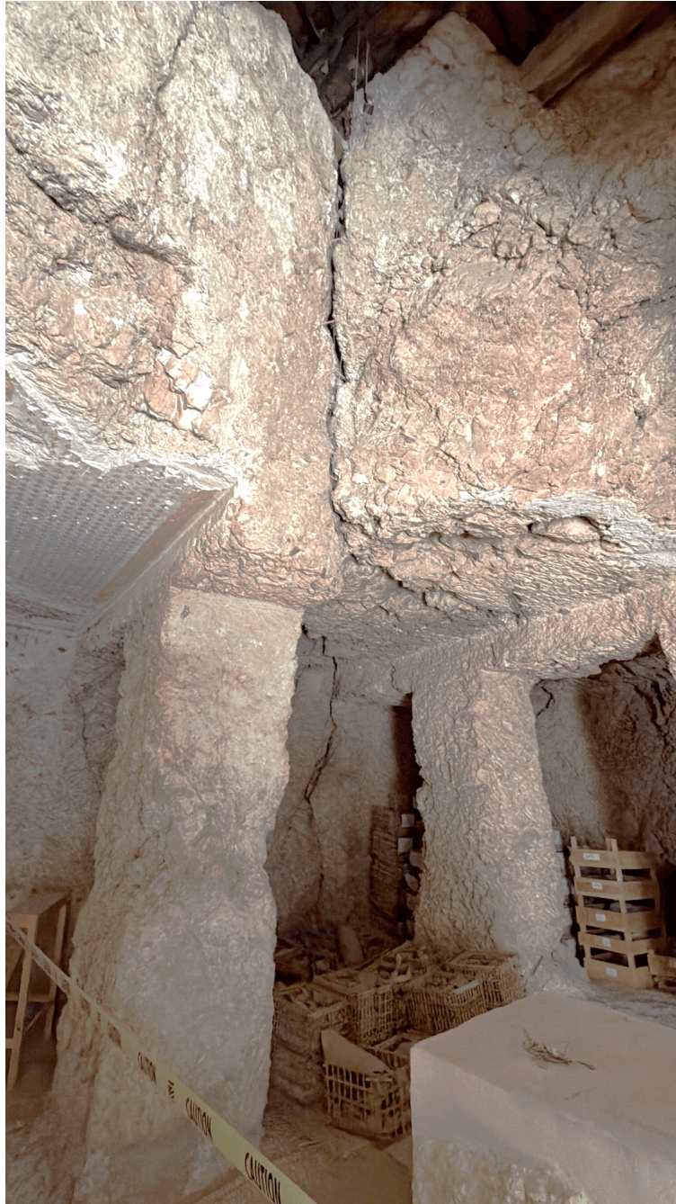
Figure 6: Image of the TT95's collapsed ceiling, assumed to be the reason why the tomb was abandoned. A constructed roof can be seen in the upper right corner. Image Credit: Bora Suda (November 2025)
