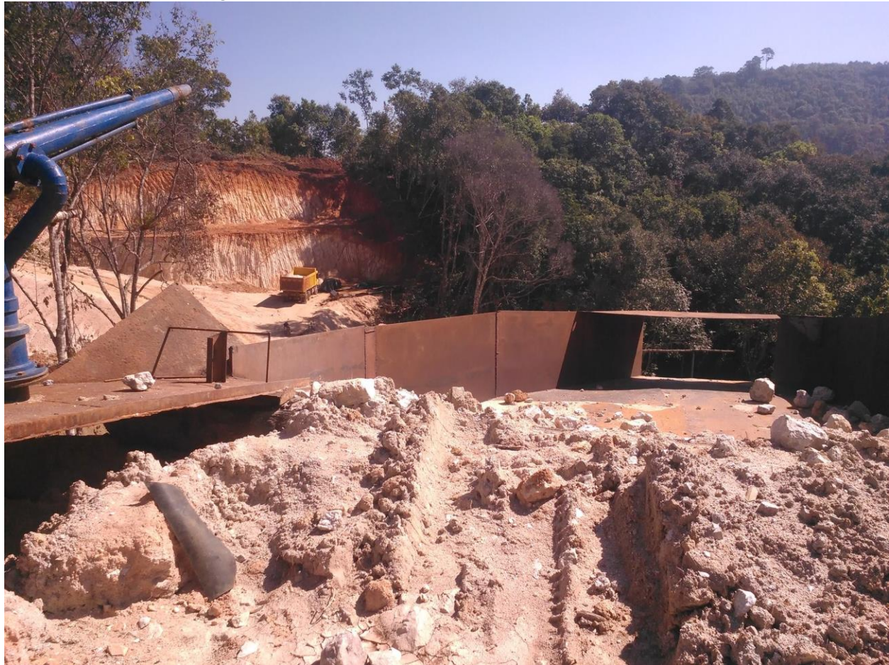
Photo 4.3. Construction at Mong Ton Dam Site. Photo Credit: Research Team, 2016
