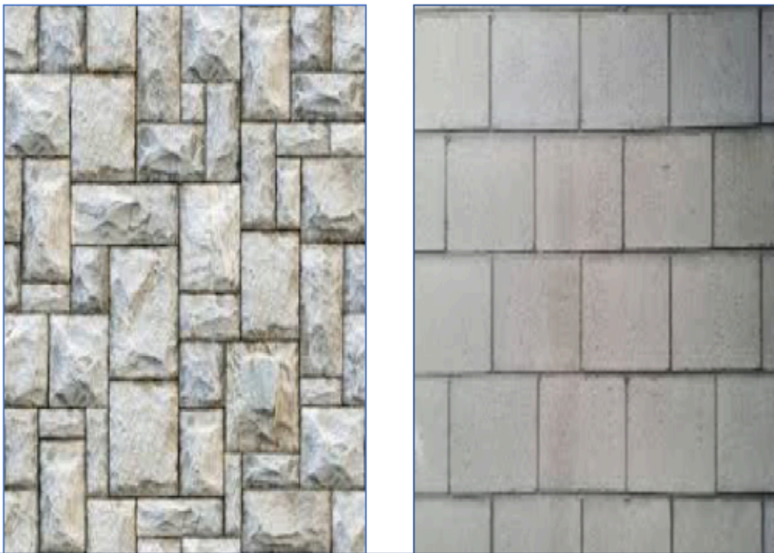
Figure 2.1) Visual comparison between the random distribution of blocks in historic masonry (left) and modern (right) construction
