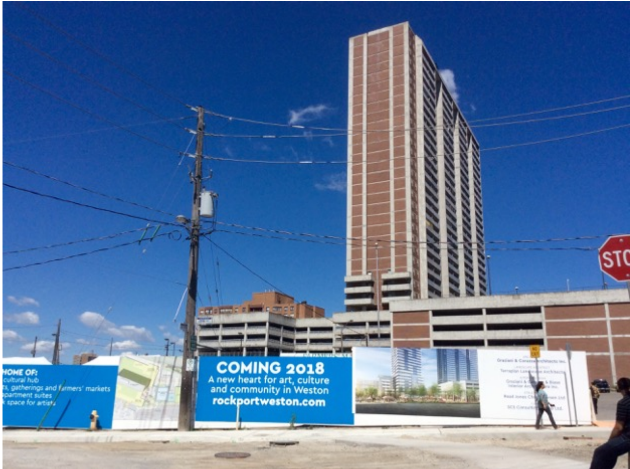
Figure 26. Construction hoarding surrounding Weston Project site the day of groundbreaking ceremony. Source: author.
