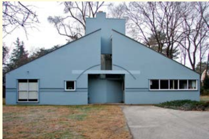
10 Robert Venturi, Vanna Venturi House , Philadelphia 1961–1964.
