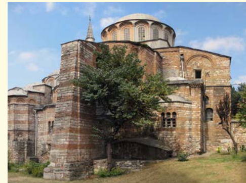
02 Chora Church, Exterior rear view, Istanbul.
