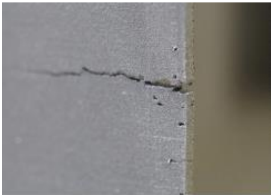
Figure 2.6 Crack Formation as a result of residual stress build-up during the manufacturing process [80]
