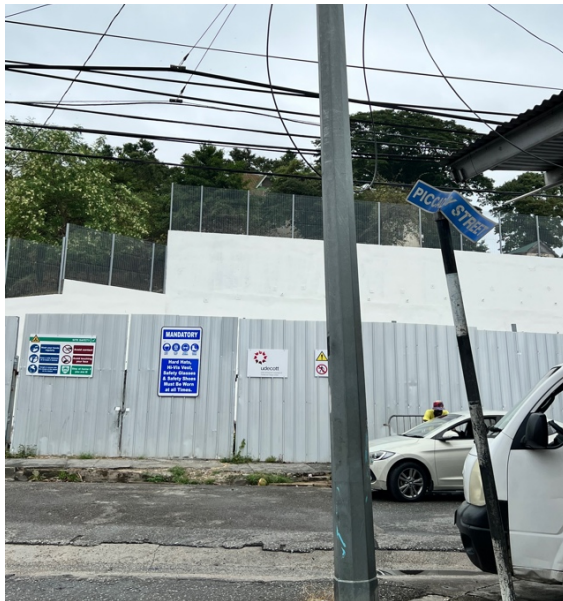
Figure 10: South view of Piccadilly Street Project Site (Source: Breanna Syne)
