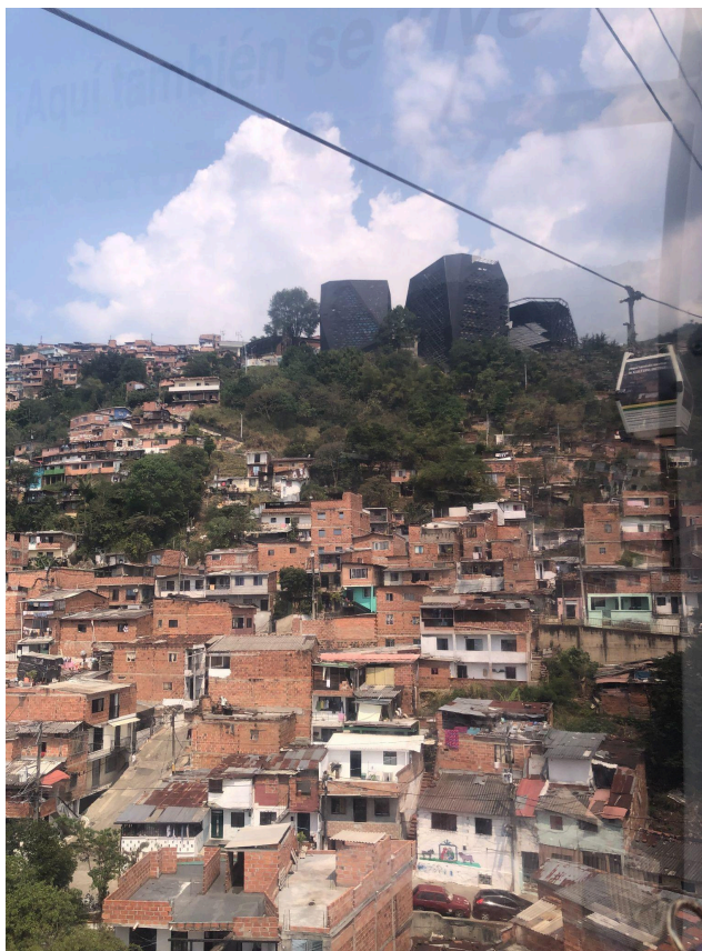
Figure 6. The Biblioteca España when viewed from lower on the hillside, demonstrating its highly visible presence. Photo by T.J. Bamonte.
