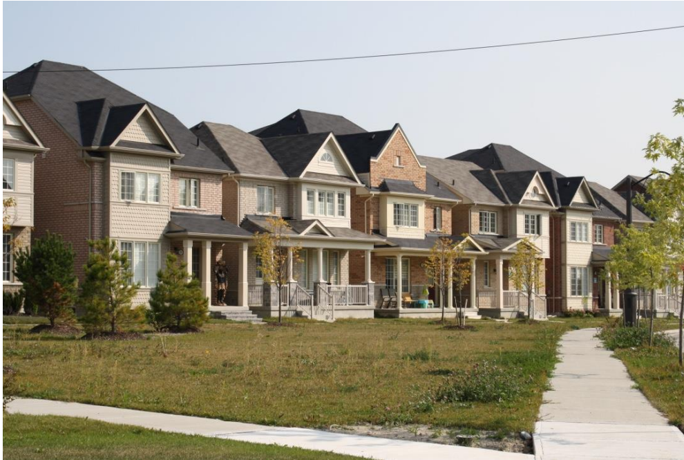
Figure 12: Single-detached homes with rear laneways. Front of homes face a common greenspace. Source: Victoria Moore (September 28, 2017)
