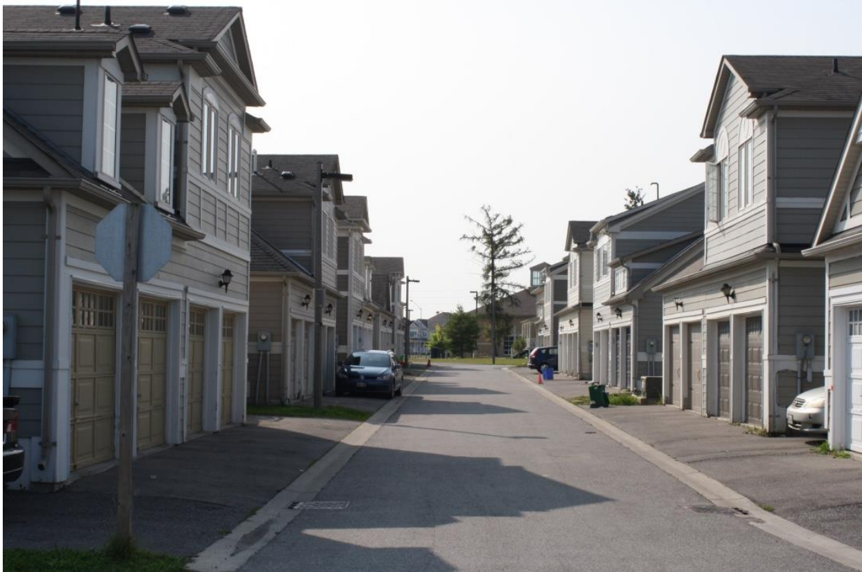
Figure 20: Rear Laneway behind semi-detached blocks with double car garages and potential coach houses above Source Victoria Moore (September 15, 2017)
