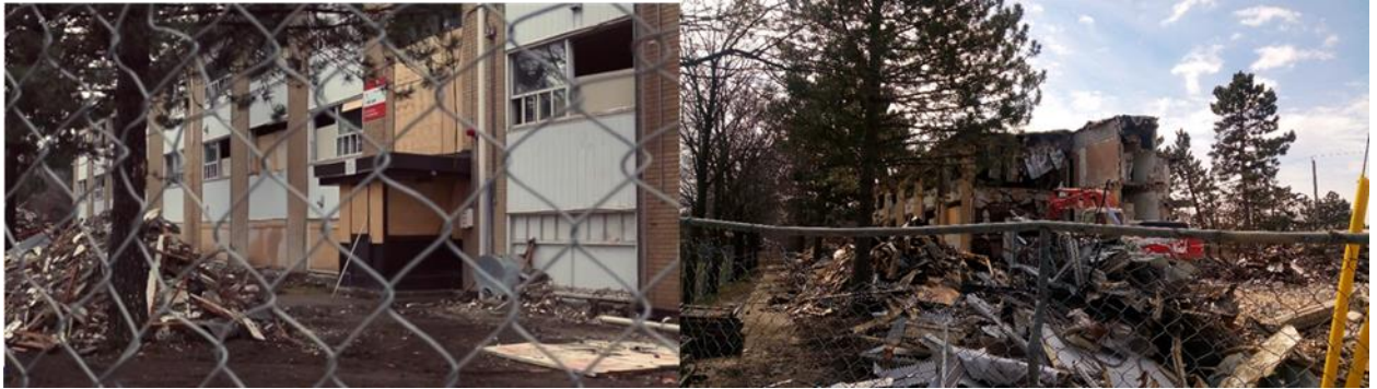
Figure 2 - Picture of 1 Leila Lane demolition site (TCHC, 2021). Reproduced with permission.
