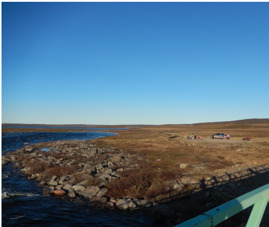
Figure 13: View of our picnic area from The Bridge. July 2, 2015. Photograph by the author.
