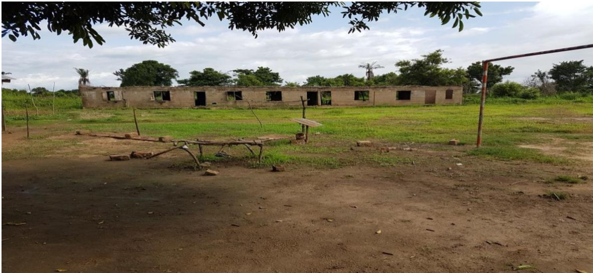
Figure 31 Remaining structure of old school left after the flooding
