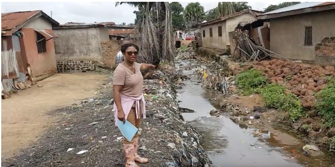
Figure 25 Residential area in Wurukum without drainage
