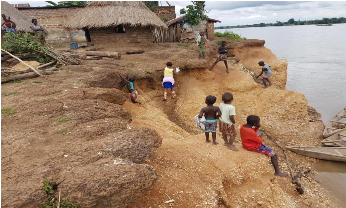
Figure 24 Hausa-Quarters, Katsina-Ala- proximity to the river
