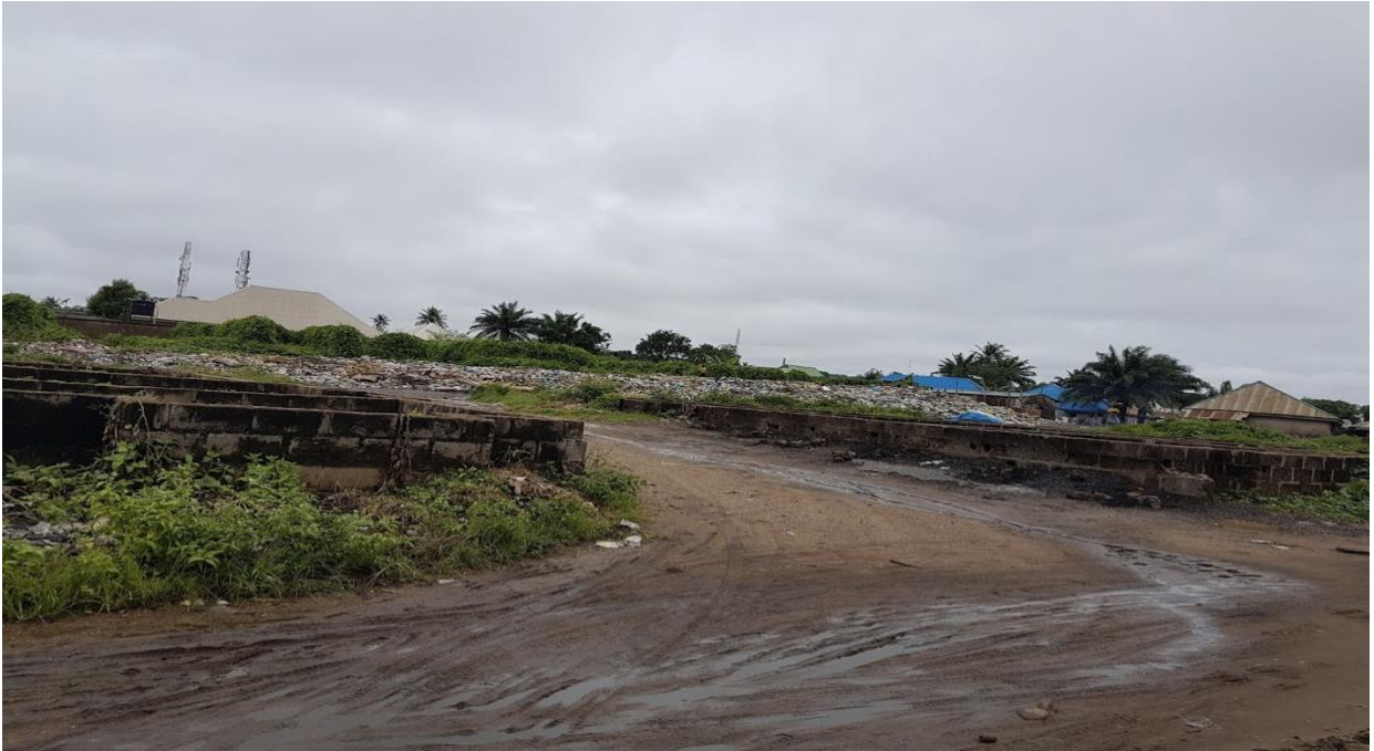
Figure 23 Waste dumping on the street causing flooding (Wurukum, Makurdi)
