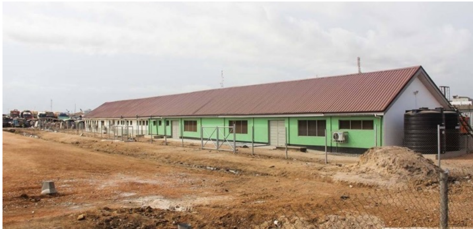
Photo 1. Completed Community Health Facility and Technical Training Centre in Agbogbloshie Source: Field assistant
