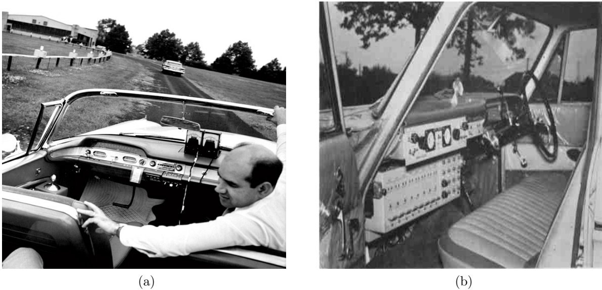
Figure 1.6: a) GM's automatically guided automobile [22] and b) Tsukaba Lab's autonomous car [23].
