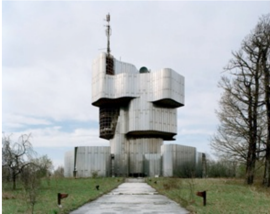
Figure 2. 20. Vojin Bakic, Monument to the Partisans , concrete, stainless steel, and glass, Petrova Gora, Croatia (view in 2010)
