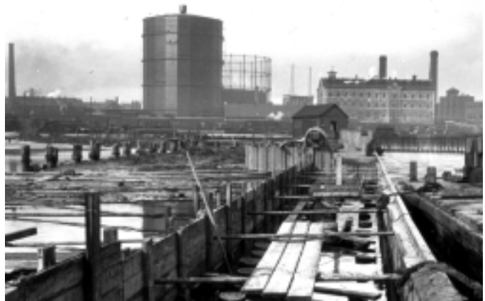
Construction of the Parliament Street Slip, circa. 1926
